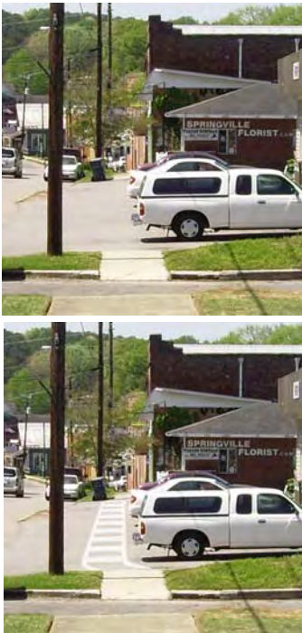
Installation of “marked” sidewalk across parking/driveway area along Main Street.
